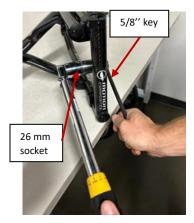
2. Tighten the nut with the 26 mm socket and finalize the installation with the torque wrench adjusted to **61 Nm**.
